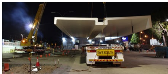
Kenwick Station composite roof 7Jun. A single piece sculptured monocoque canopy designed for durability and rapid overnight installation. Capital House Australasia Perth, made by Swarbrick Technologies. Image courtesy B Nelson
