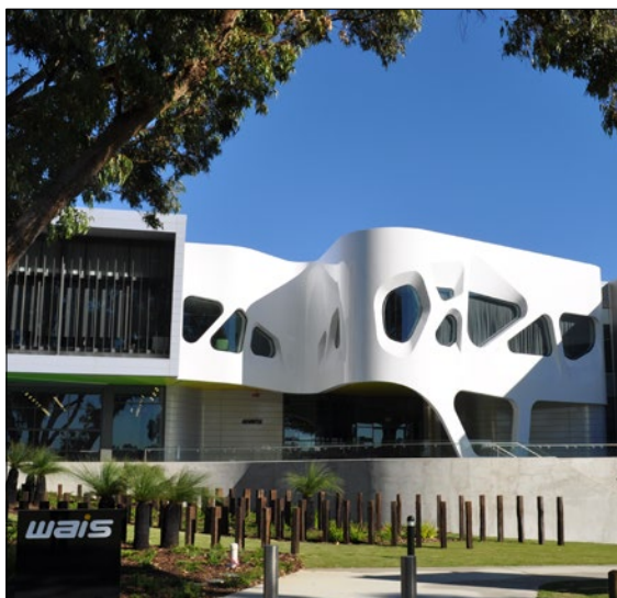
Western Australian Institute of Sport (WAIS) composites facade. Architects, Sandover Pinder with Melbourne partners dwp/sutars architects, made by Swarbrick Technologies in Henderson and transported to site. Image courtesy WAIS.
